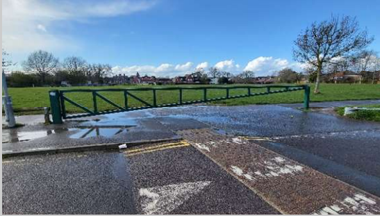
Figure 2 – Kings Centre car park vehicle access barrier
